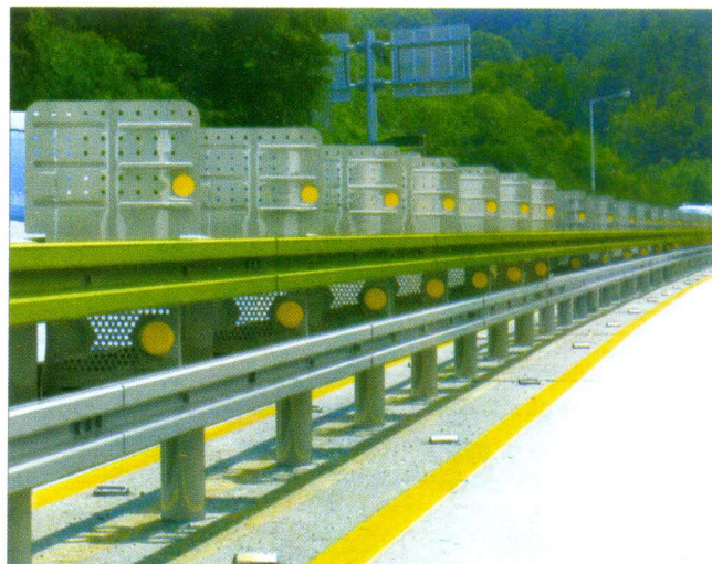
[ Photo showing assembly of rail+rail stiffening plate+glare shield ]
