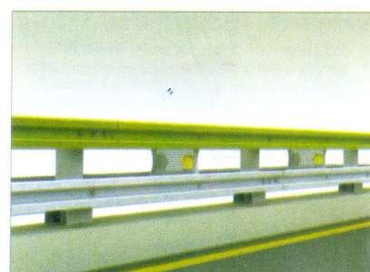
[ Assembled View of Rail and Rail Stiffening Plate ]
