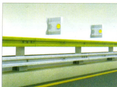
[ Assembly of Rail and Rail Stiffening Plate ]
