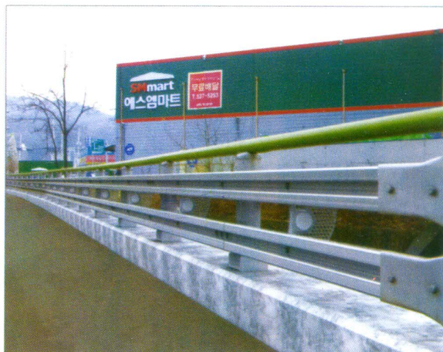
▲ APocheon city Bupyeong-2gyo of 2 steps x L2,000F-SBGrade5
